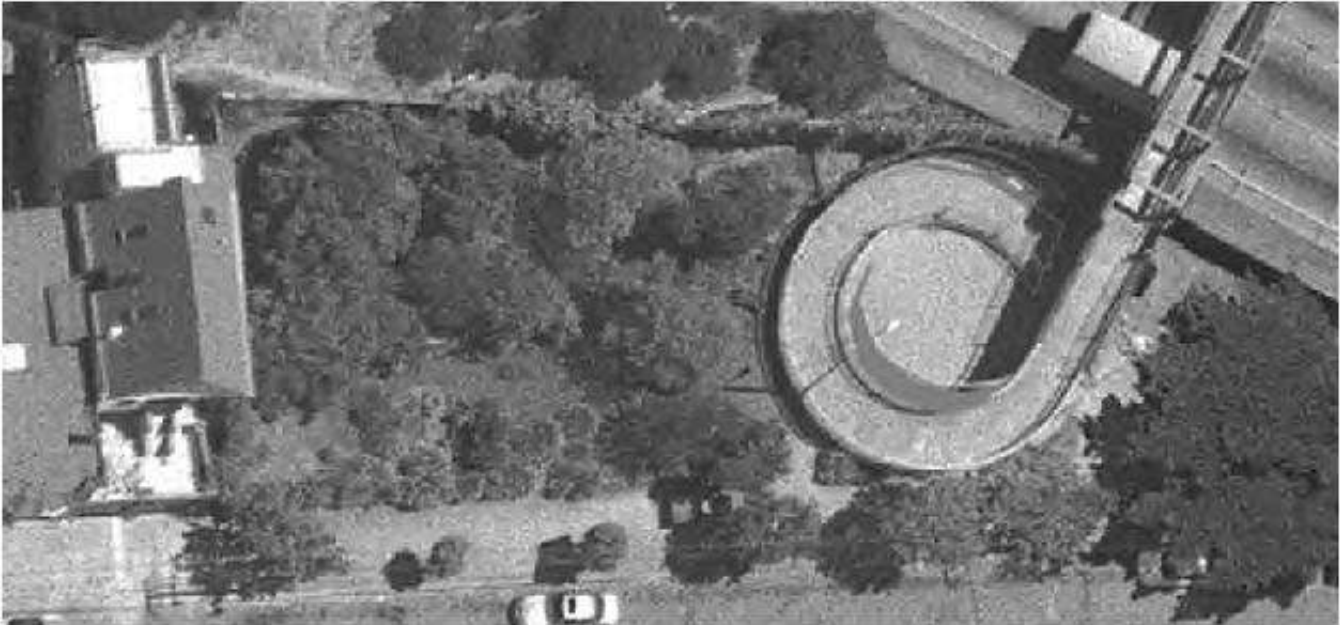
Ariel View of Fallen Bridge Mini-Park
